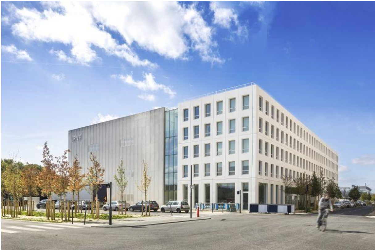
Figure 3 - The IPVF building
