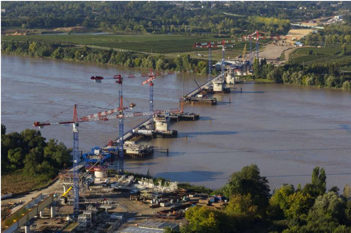
Figure 11 - The construction site of the Dordogne bridge
