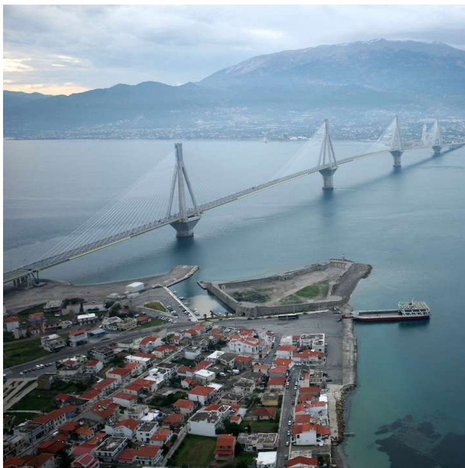
Figure 9 - The Rion-Antirion bridge
